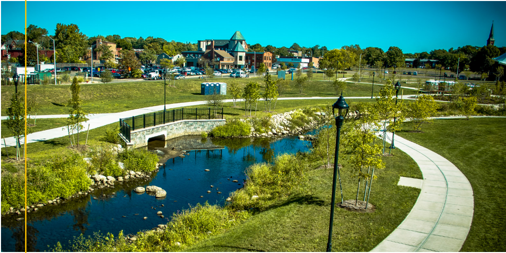
The Meriden Green, a 14-acre flood-control park in Meriden, Connecticut. Photo source: Marcus Balcher, Meriden resident
