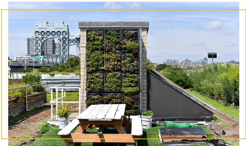
A green roof on the NYC Parks Department building on Randall's Island. Source: NYC Parks
