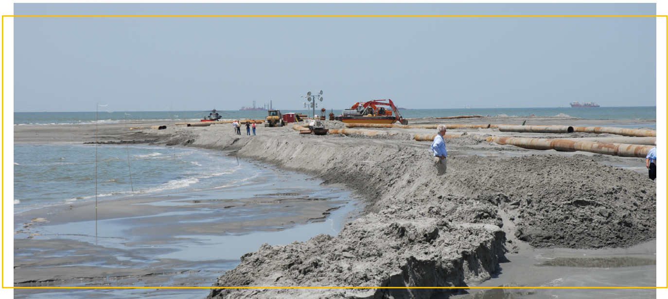
Dredging and sand berm construction coastal Louisiana protect Louisiana's marshlands.
