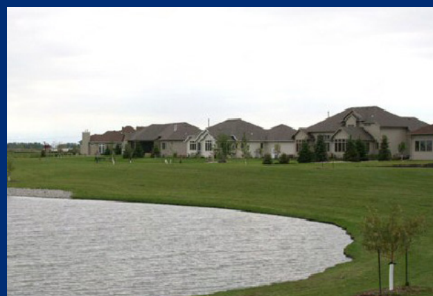
Woodhaven in Fargo, North Dakota, has a large stormwater retention pond that collects stormwater runoff and drains it into an underground aquifer slowly, filtering the water in the process.
