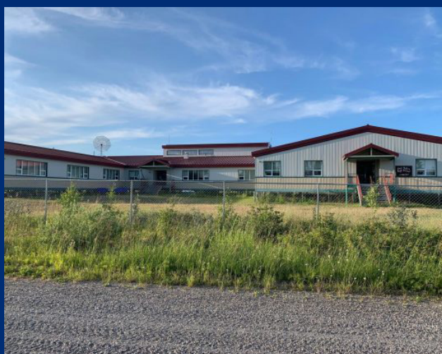
Pictured above is the schoolhouse in Fort Yukon, Alaska. In 2018, $1 million in HMGP was used to raise 9 structures onto stilts. Source: Alaska Public Media
